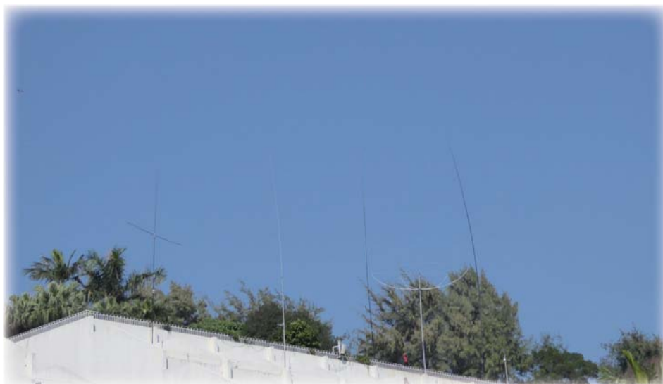
Our antenna farm on the 8 th floor
