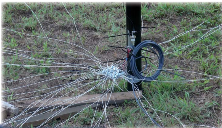
Base of 160 meter inverted-L
