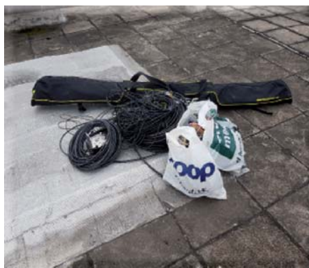
ALL antennas wires and cables
