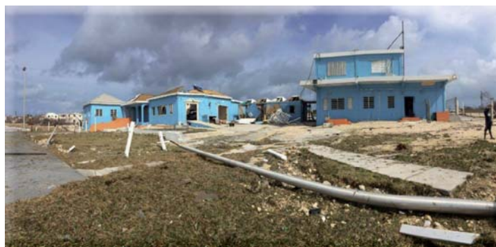
Blowing Point Ferry Terminal.
