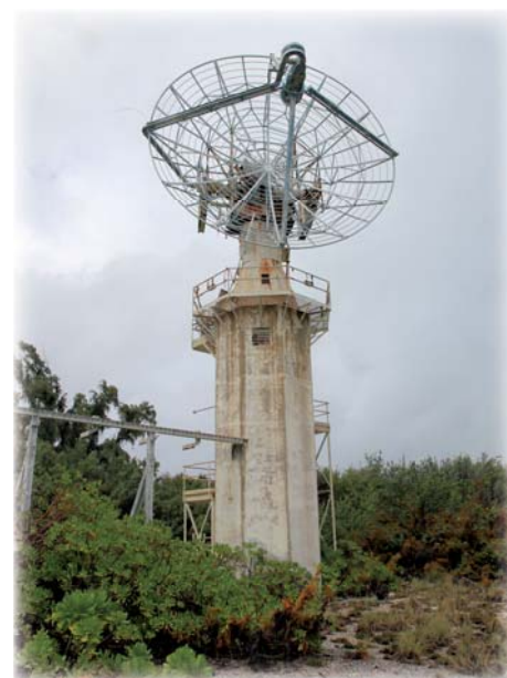
Old satellite station
