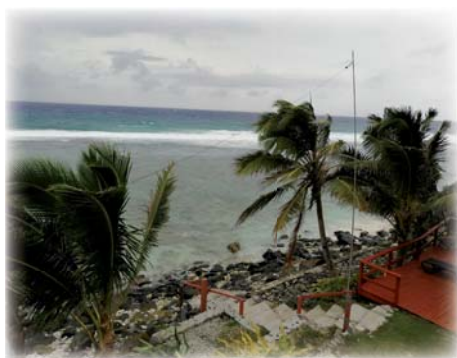
The antenna built up at the coastline
