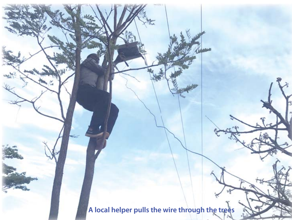
Vasily, RA1ZZ, installing the beverage RX antenna
