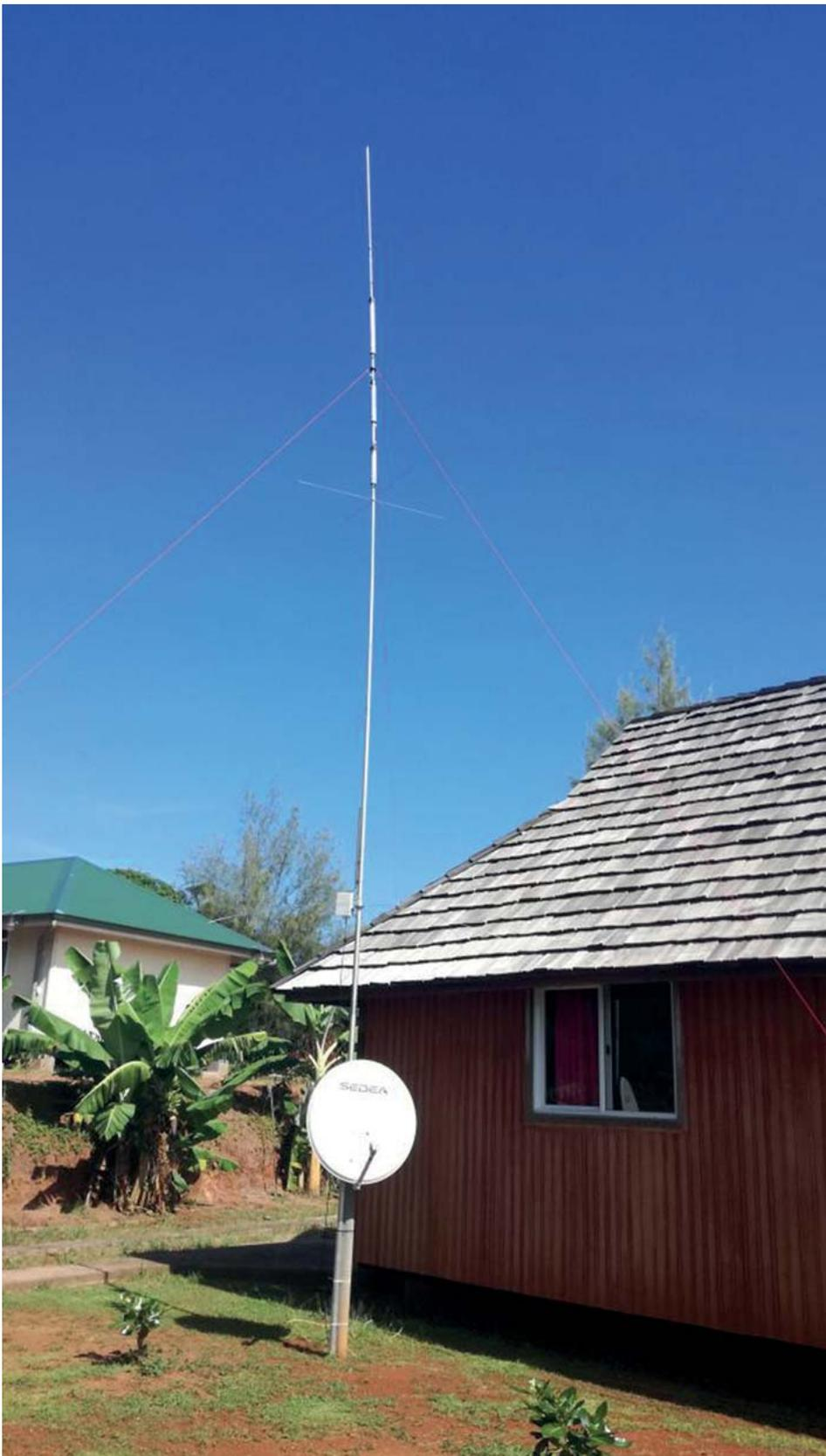
In the morning after arrival, I installed the multi-band vertical, and a few days after a delta-loop for 80 m supported in the middle by a 12 m Spiderbeam mast. The vertical was fixed to an unused satellite TV mast.
